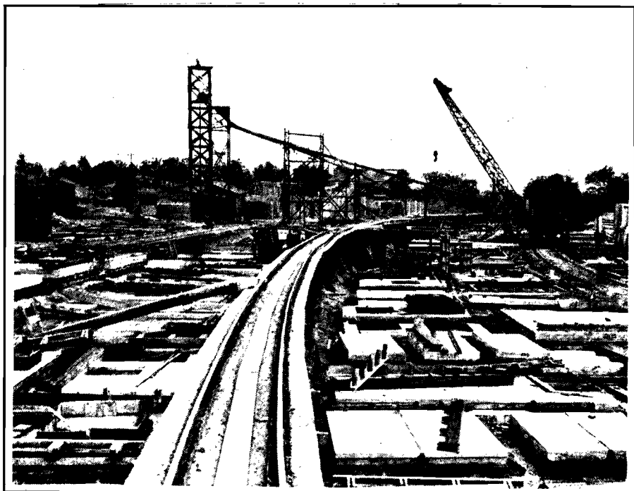
Fig. 4. General view of casting yard. Note the trestle track running from the central concrete plant through the yard.
